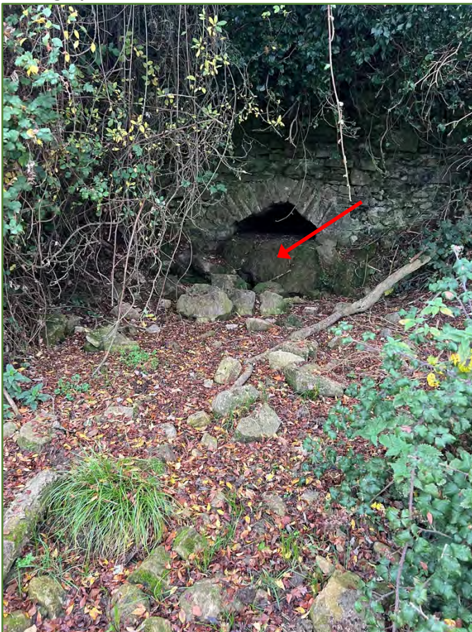
Photograph 3. Culvert under road with old cascade tufa formation (view to south)
