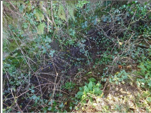
M19 – base of drain that “flows” between N19-N18; damp, slick mud with no fisheries value.
