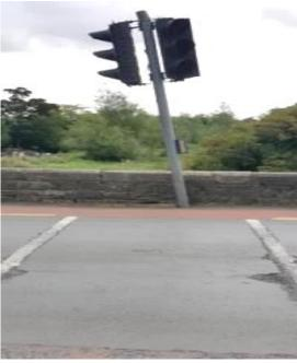
Figure 2.11: Examples Showing Damage to Traffic Signals at The Square and Slane Bridge
