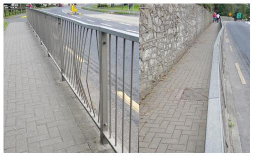
Figure 2.8: Damage to Pedestrian Guardrail in Slane Village
