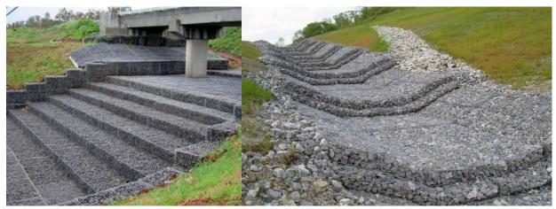
Figure 3.15: Examples of Gabion baskets and Reno mattresses
