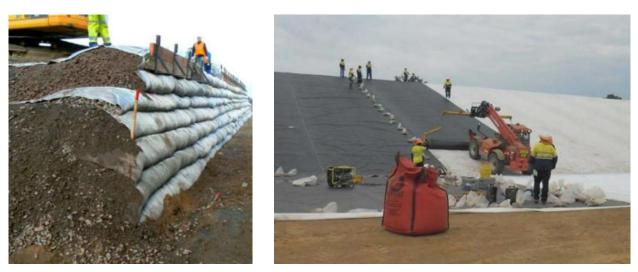
Figure 3.10: Typical Arrangement of Geotextile Placement / Wrapping
