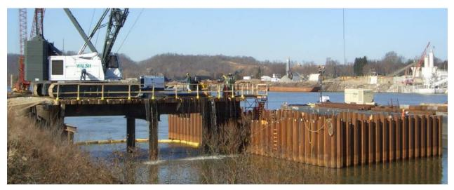
Figure 3.16: Example of Coffer Dam
