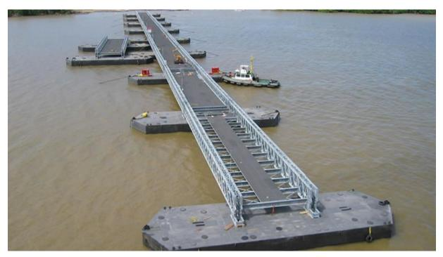
Figure 3.14: Example of Bailey Bridge with Pontoon Piers
