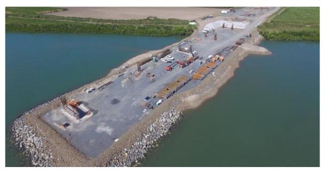
Figure 3.12: Typical Arrangement of a Bunded Working Platform
