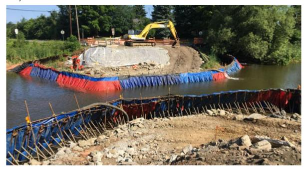
Figure 2.4: Example Cofferdam<sup>3</sup>
