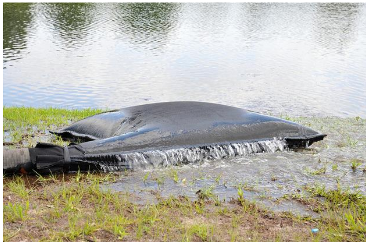
Figure 5.3: Silt Dewatering Bag
