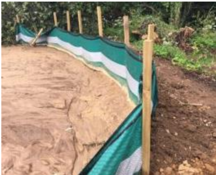
Figure 5.4: Typical Silt Fence
