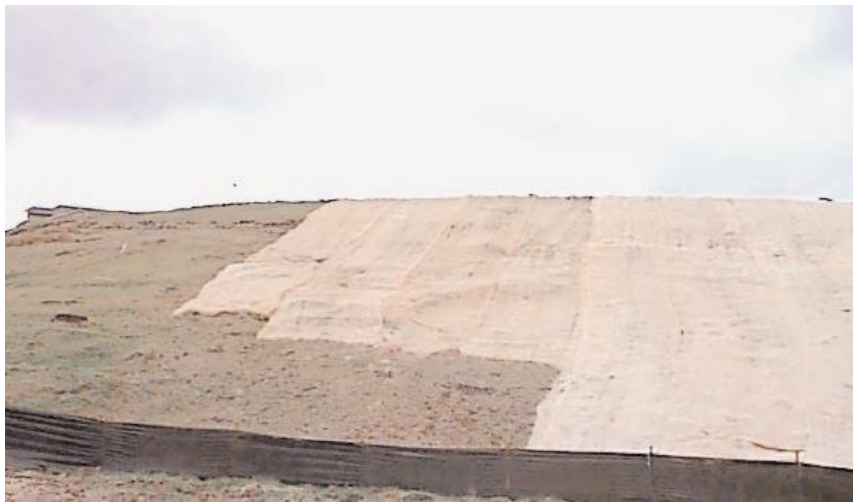
Figure 5.2: Coconut matting on earthworks slope (CIRIA C648)
