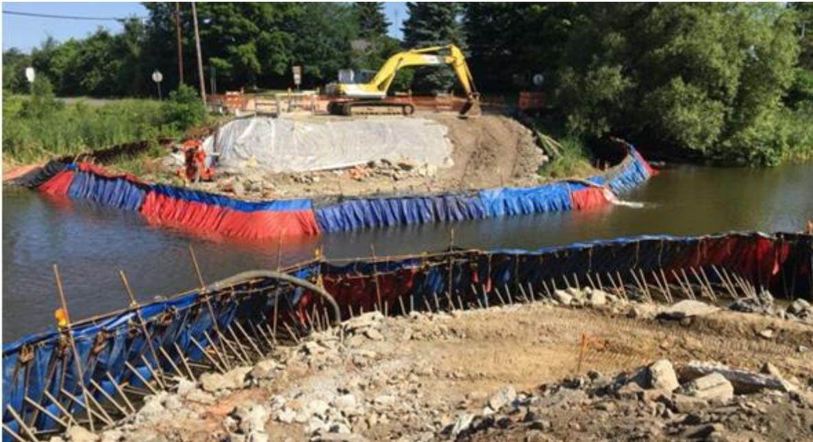
**Figure 5.2: Example Cofferdam<sup>3</sup>**
